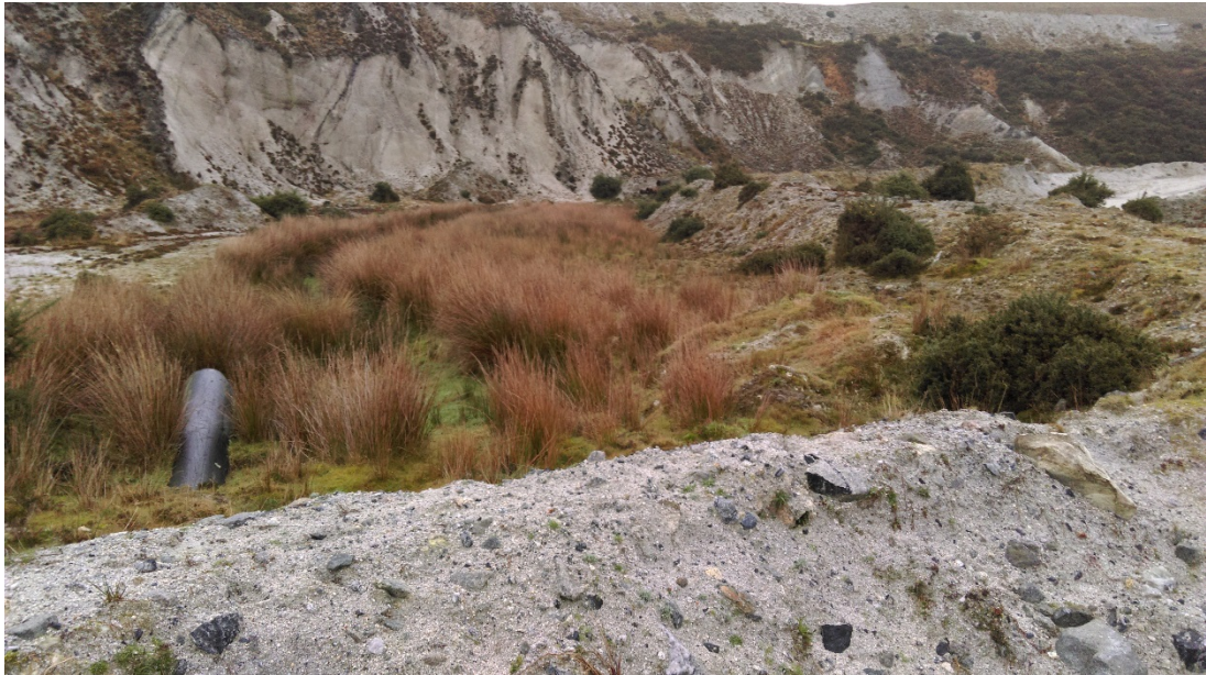
Figure 11 – Whitehill Yeo Pit – Potential area for de-watering plant
