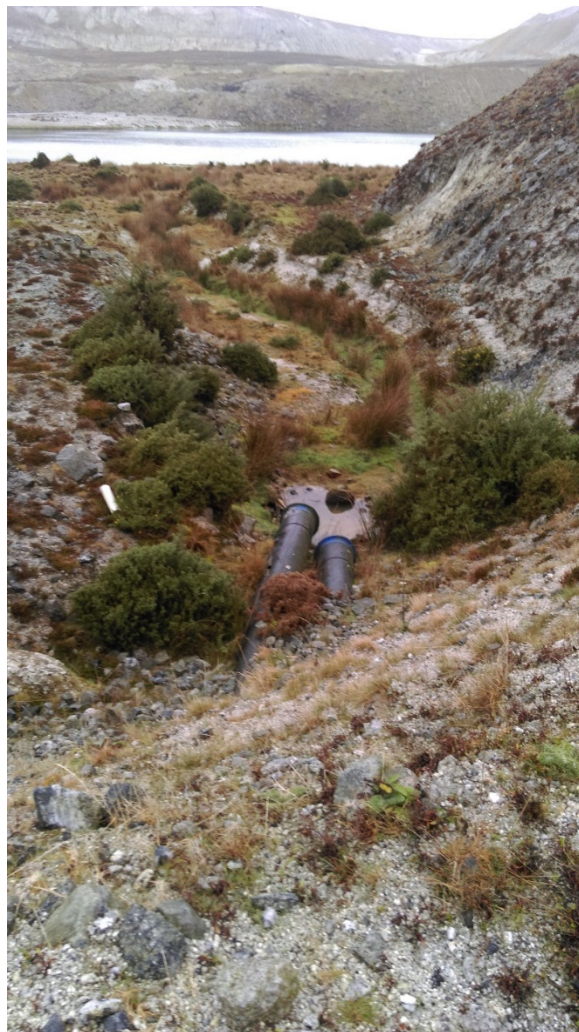
Figure 12 – Outgoing pipe from dewatering plant to launch site
