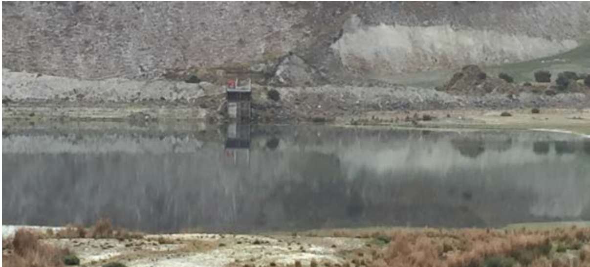
Figure 5 – Whitehill Yeo Pit South Pool – showing outlet gate on South bank
